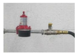
Lower gas connection to 1/2" with high-pressure regulator.
