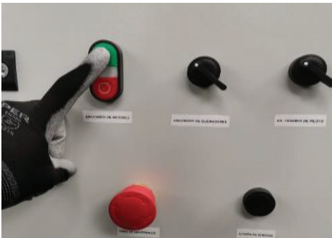
C Press green button (ON) motor ignition
